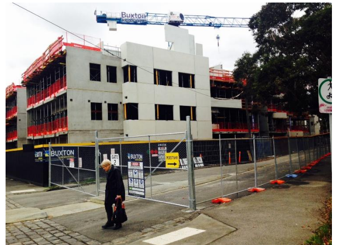
Upper level construction
