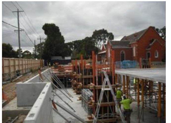
Lower Level Construction
