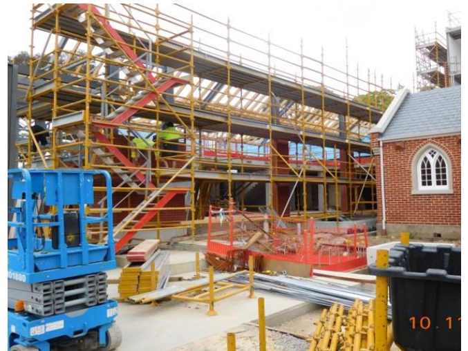
Upper level construction
