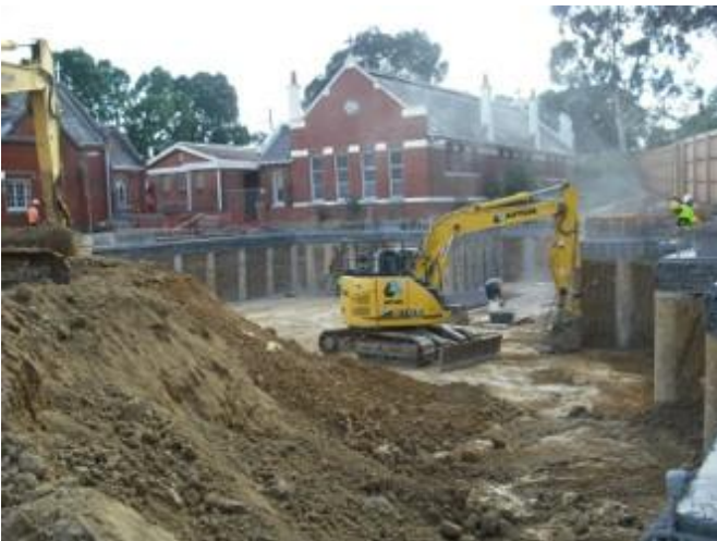
Excavation for Carpark
