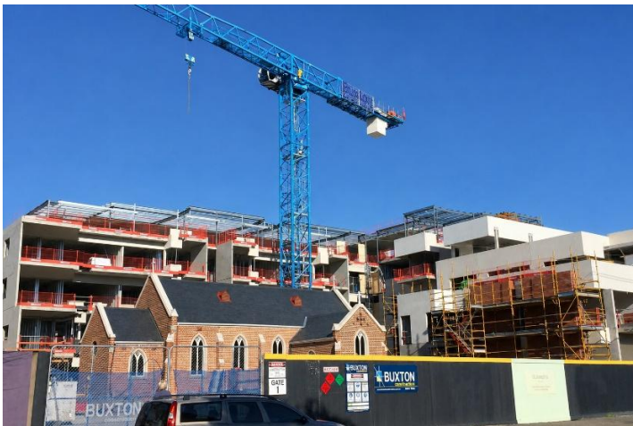
Upper level construction
